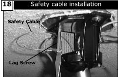
For Canadian installation and for USA fan and light kit combinations over 35 lbs, in both flush and downrod mode the safety cable must be installed into the house structure beams using the 3" lag screws provided. Make sure that when the safety cable is fully extended the leadwires are longer than the cable and no stress is placed on the leadwires.
